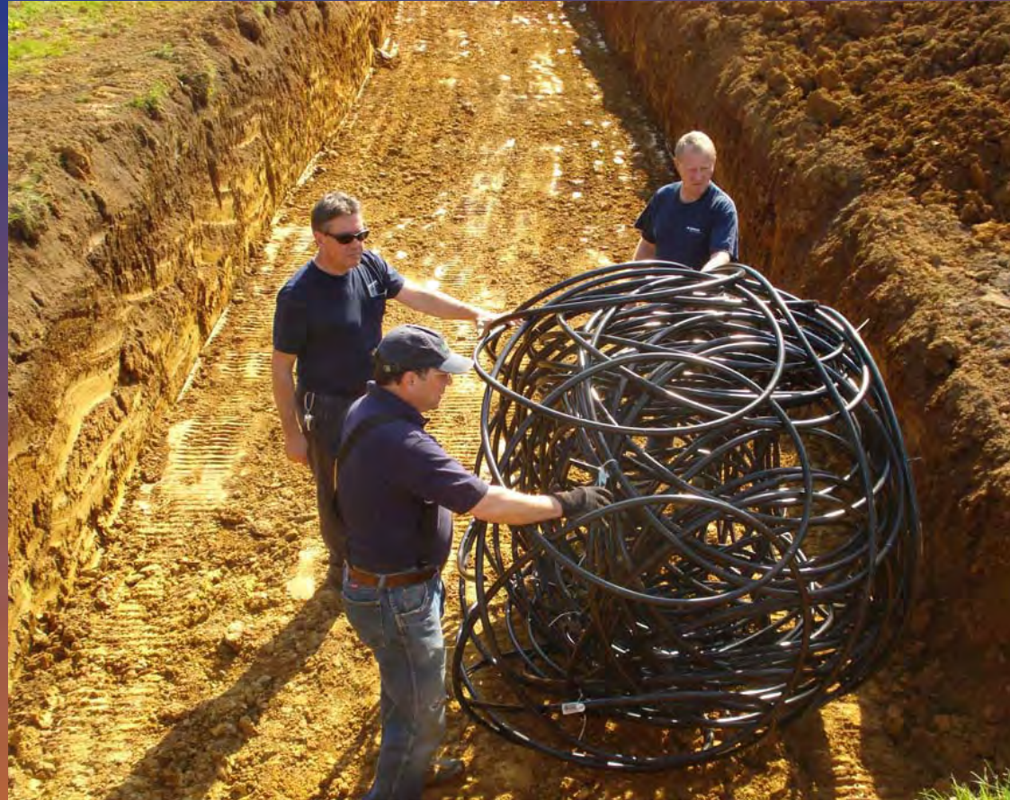
TeraTherm Horizontal Closed-Loop Pre-rolled slinky is positioned
