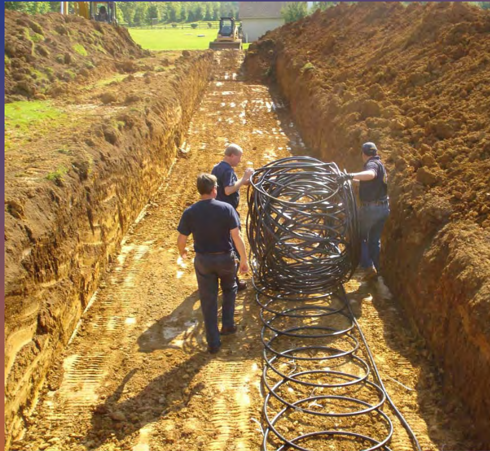
TeraTherm Horizontal Closed-Loop Pre-rolled slinky is rolled out
