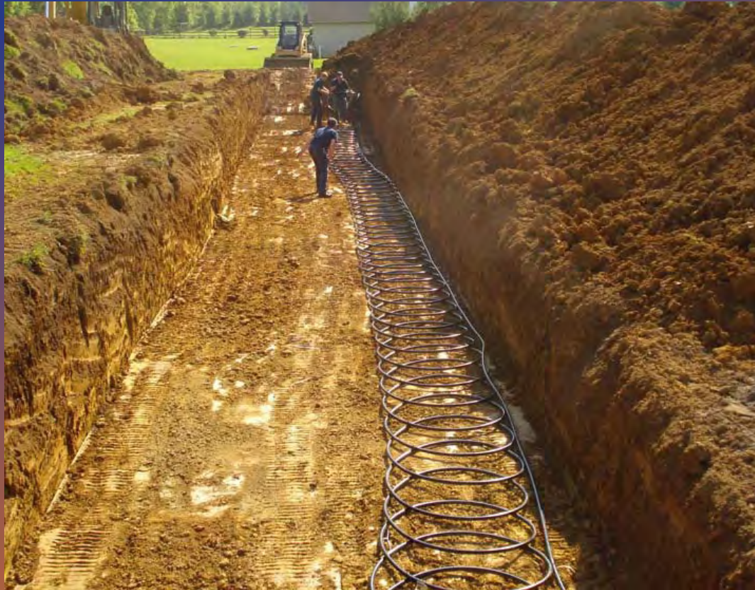
TeraTherm Horizontal Closed-Loop Pre-rolled slinky is rolled out
